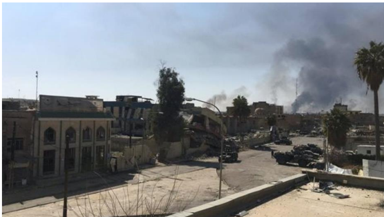
Image - A destroyed government building in the west of Mosul.
